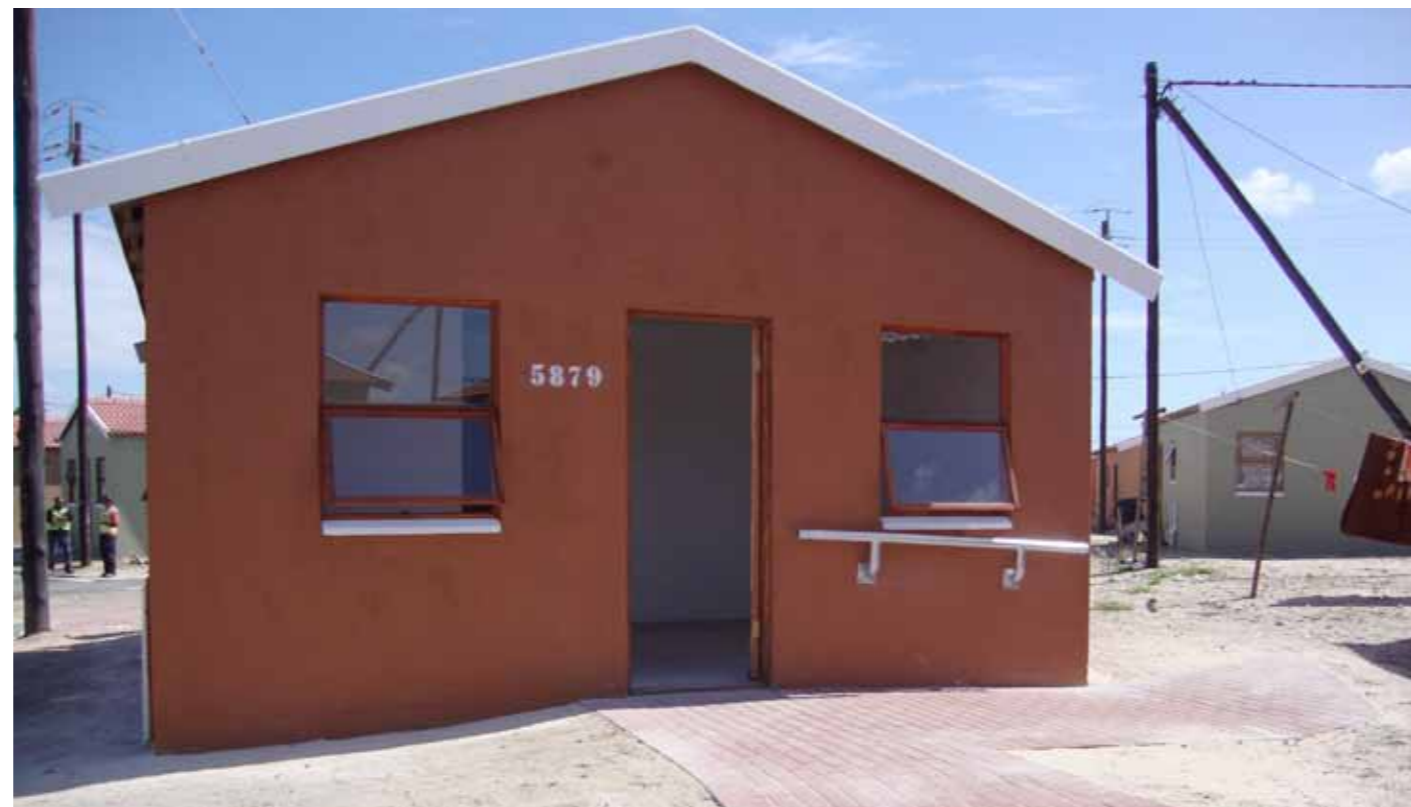
An example of a special needs house in Boystown. It is fitted with a rail along the wall and has a concrete ramp to make movement from the street to the front door easy for a wheelchair user.
