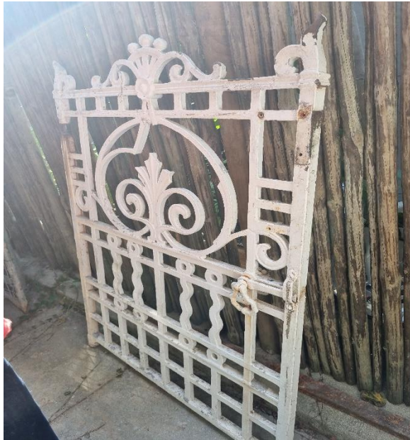
Figure 2 – Original cast-iron fence
