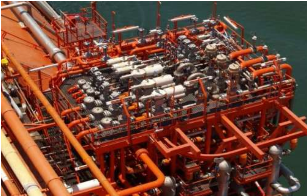
Figure 2.6 Example of a regasification unit on board of a FSRU
