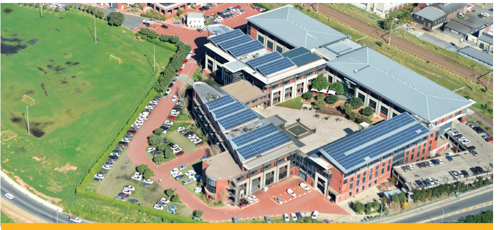
Grid-tied PV system at Black River Park.
