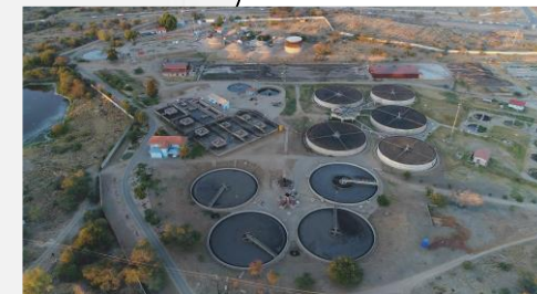
Waste digester facility
