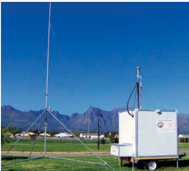
AMBIENT AIR QUALITY MONITORING STATION LOCATED AT AN IDENTIFIED AREA SOURCE.
