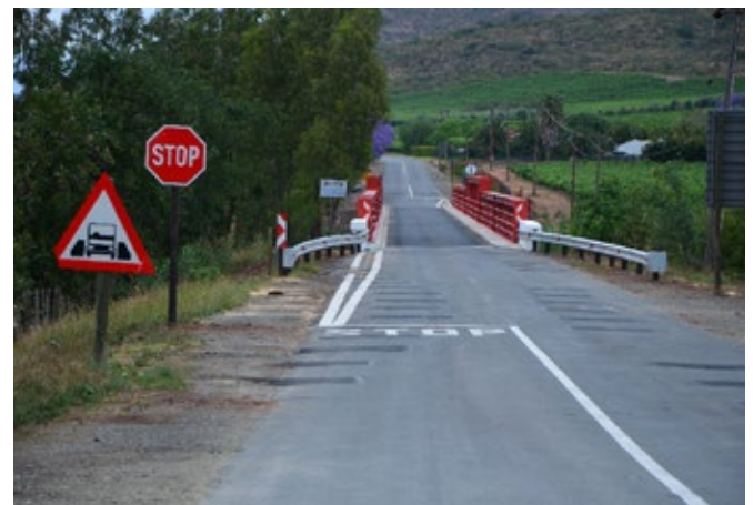
The bridge after the work was completed.
