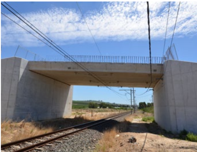
The construction of a pedestrian footbridge at Lynedoch Station.
