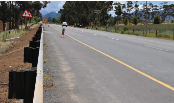
Installation of new guardrails on both roads.
