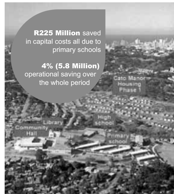
Photo 14. Facility Clustering Cato Manor, Durban (CMDA)
