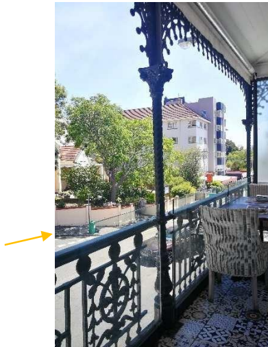
Fig.2 Frameless glass at first floor balcony can hardly be seen.
