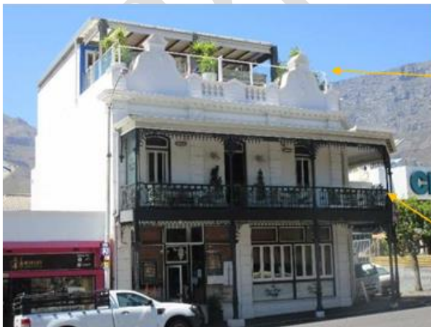
Fig.1 View of the Kloof Street elevation – note visible steel supports and railing installed at ‘frameless’ glass behind the distinctive parapet.
