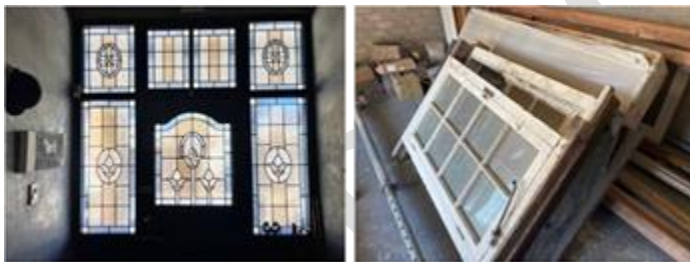
Left: Good surviving leaded glass front door. Right: Casement windows recovered from the building and stored on the first floor.
