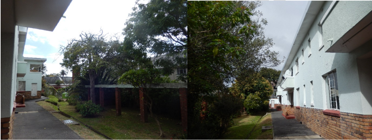
FIGURE 1 B: Back façade of Werverdiend (22 Rouwkoop Road)
