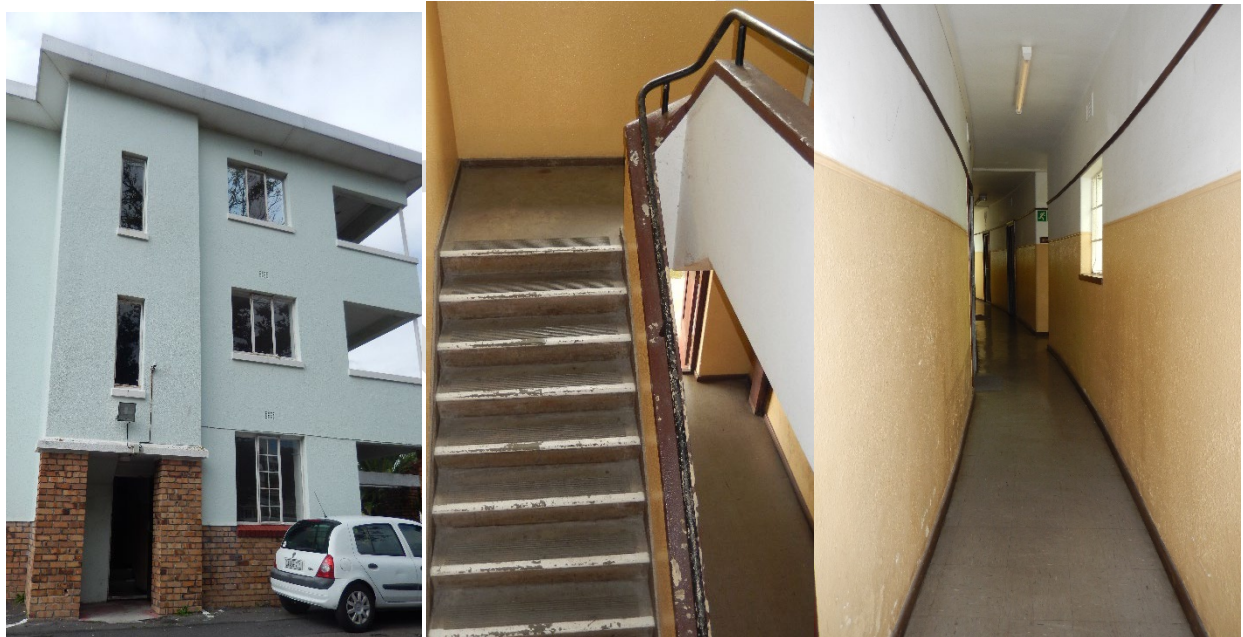
FIGURE 3: Narrow entrances, staircases and corridors
