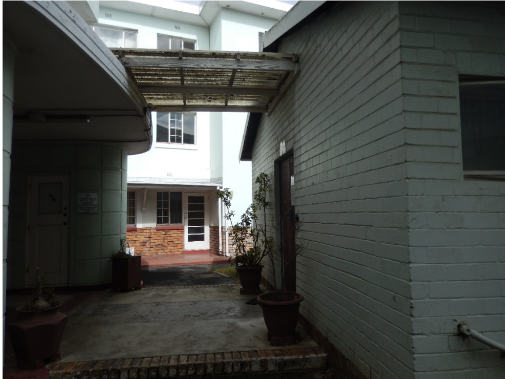
FIGURE 2: Additions to the main structure
