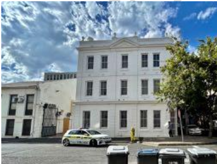
FIGURE 01: The corner building which is to be retained (centre) with a portion of the former NICRO building to the left.
