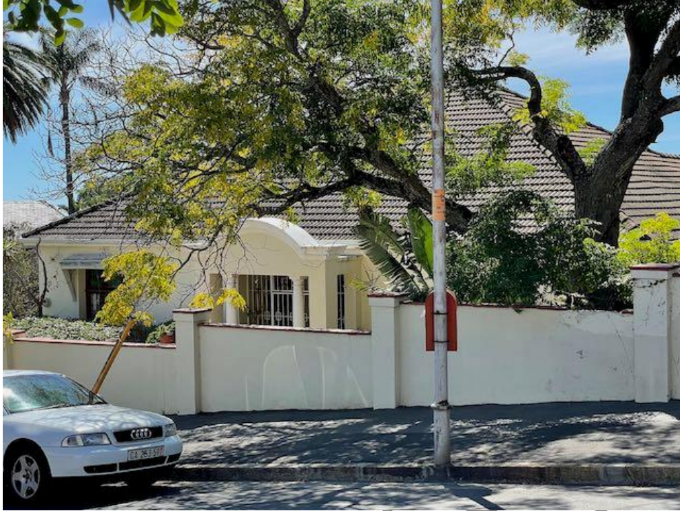
FIGURE 04: The neighbour on the uphill side: architecturally similar to the house in question.
