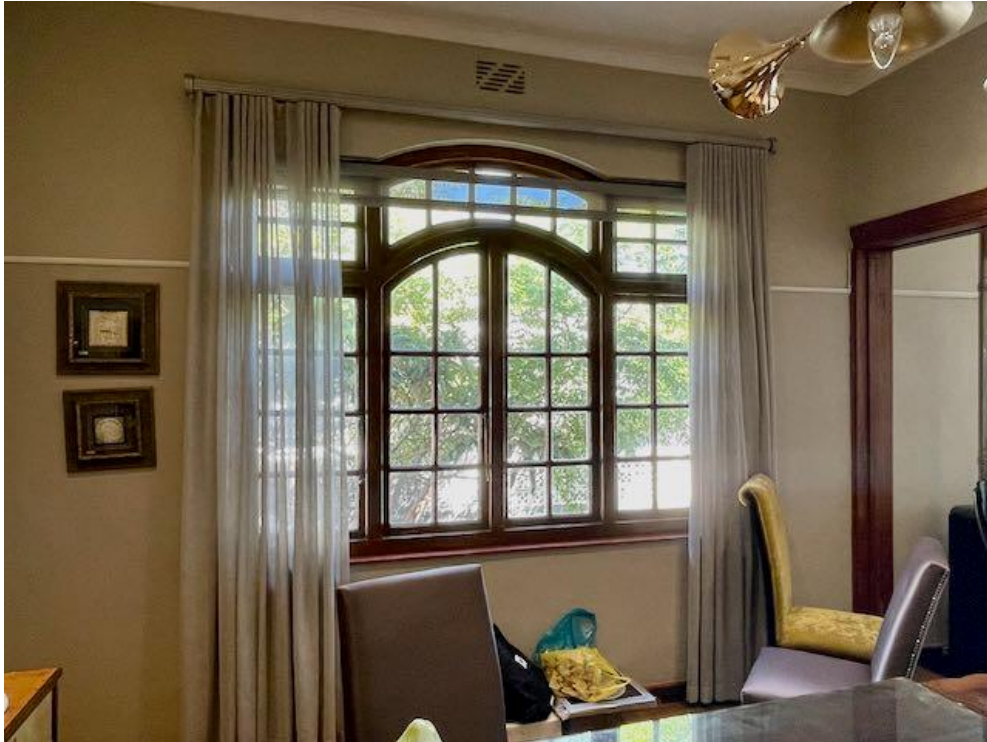
FIGURE 07: Good surviving 'modified Palladian' casement window in the living room.
