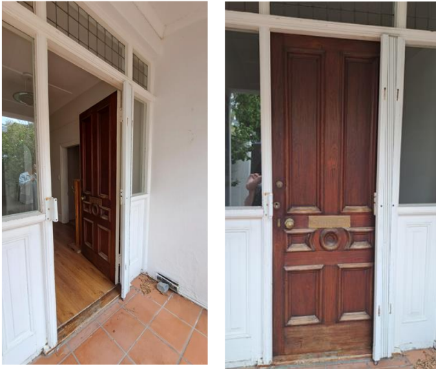
Figure 16 & 17: Detail views of teak timber entrance door with lead fanlight and side lights
