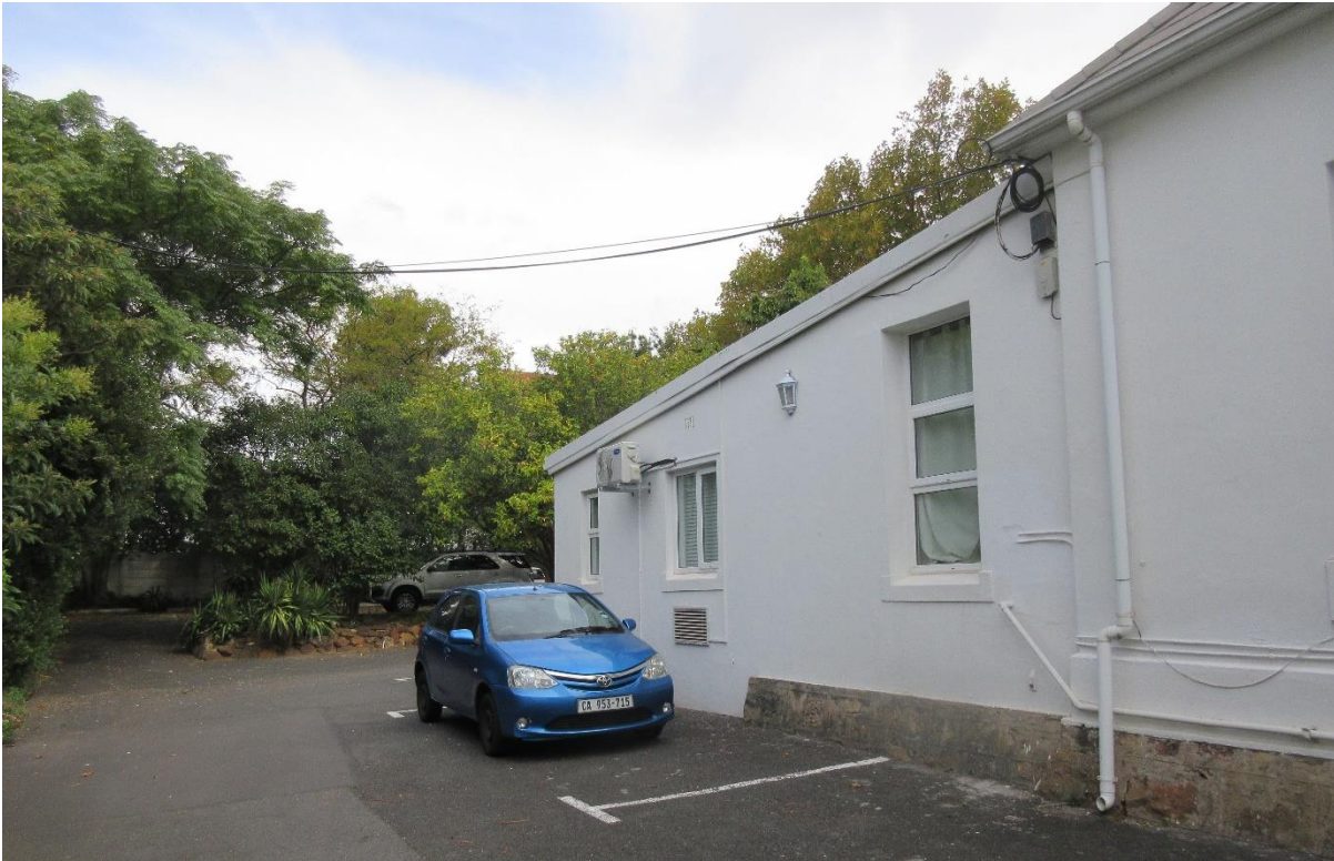
The original building had been extended southward yet still left a large portion of the site open for parking.
