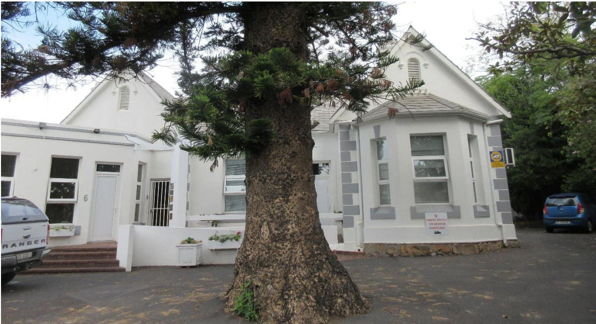
The subject building on 6 Kenilworth Road, seen from north.
