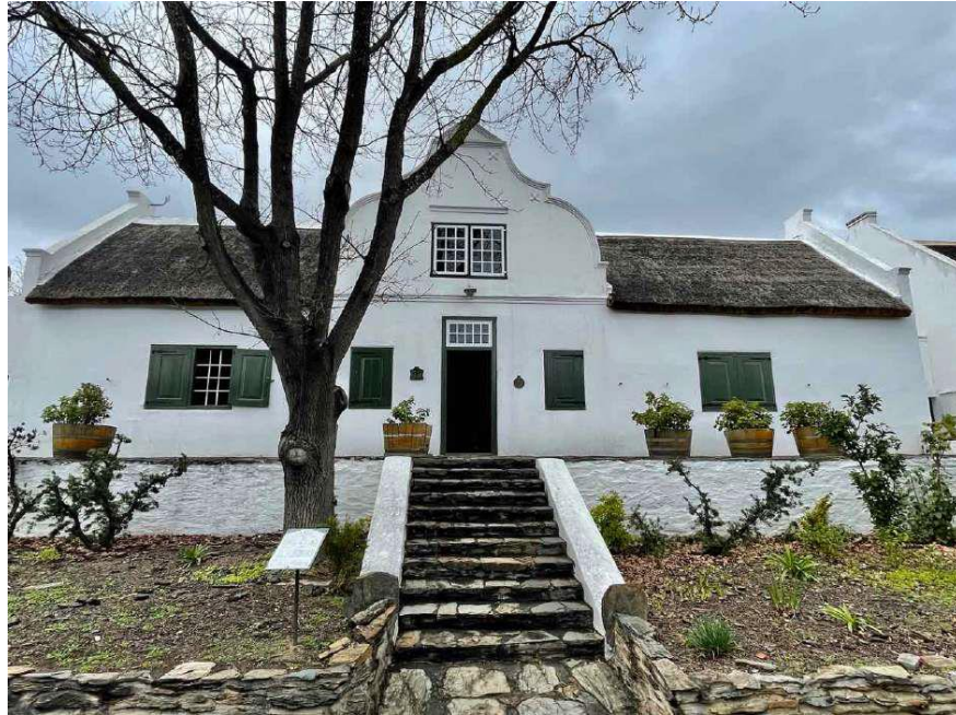
The front of the house facing Church Street (not affected by the unauthorized work).
