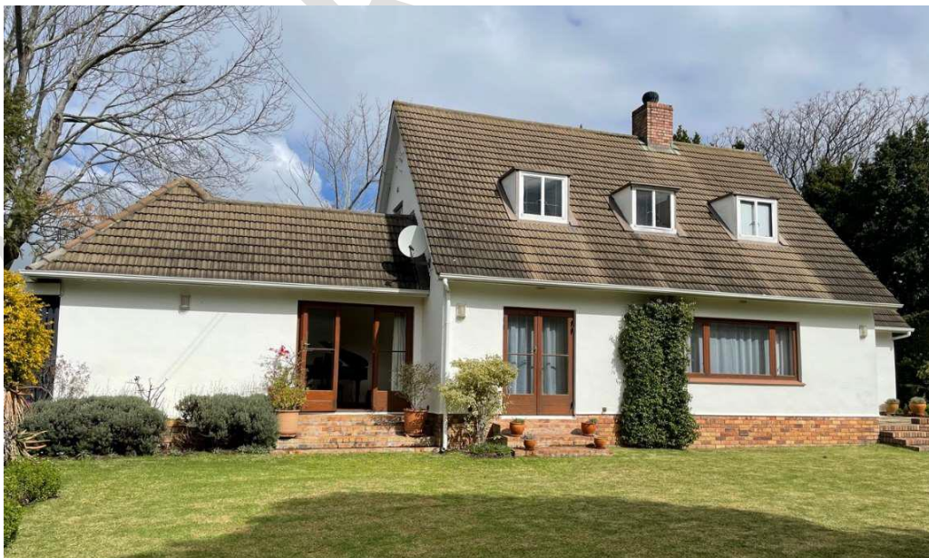
The double-storey, central portion of the north elevation to the right of the image. Different from the two hipped dormers shown on the original plan, three were realized but with flat, horizontal roofs, and gutters on three sides, a want of eg CFA Voysey, see his Broadleys. The waterproofing is of copper dressed to best practice.
