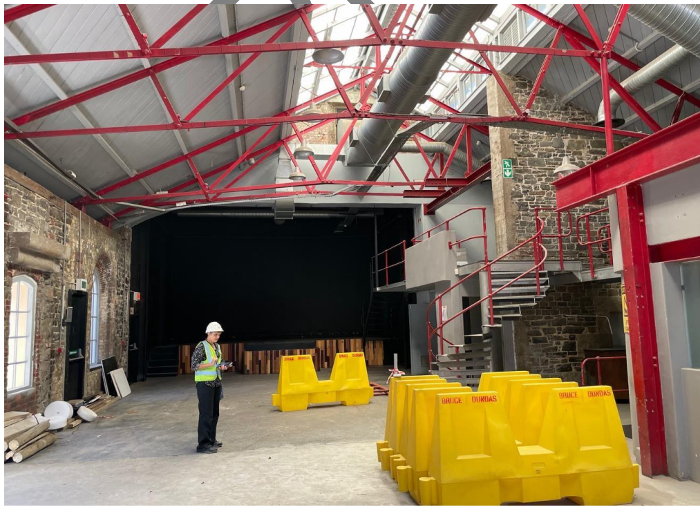
Figure 6 – Interior of the Pump House Building
