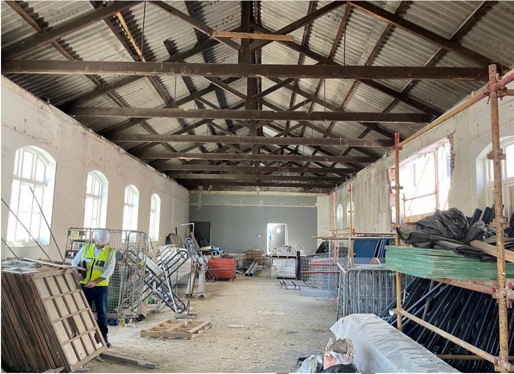
Figure 3 – Interior of the Forum building, with various items being stored.
