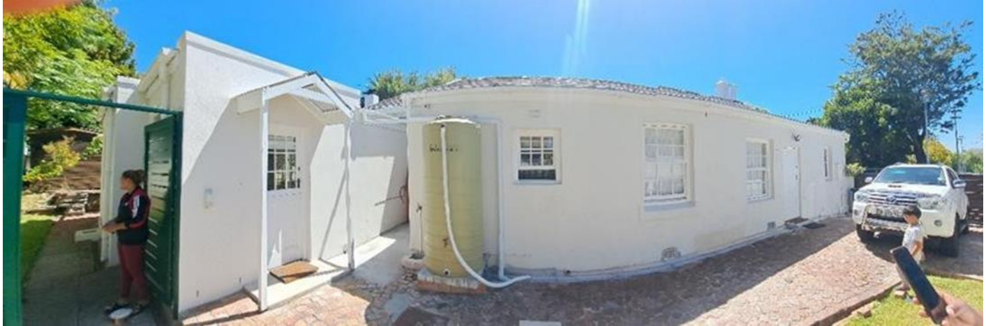
Figure 3: South elevation with the adjacent space to be converted to a double carport.
