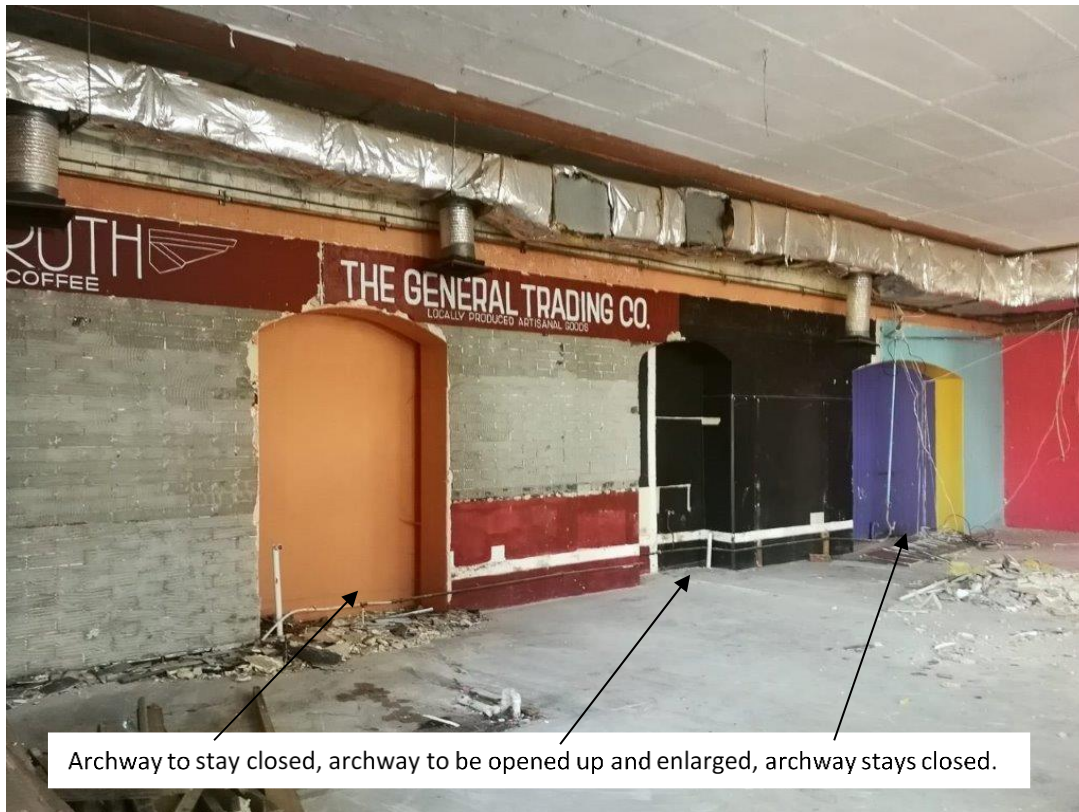
Figure 5 – the wall separating the Power Station from the Pump House, the central archway to be opened up and enlarged (to detail being awaited by HWC).
