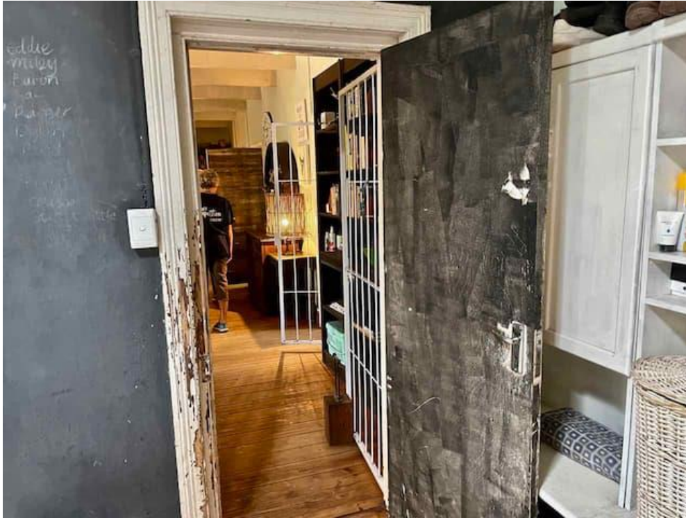
FIGURE 06: Latter 19th/Early 20th C moulded timber architraves with flush doors which are replacements. (Originals would likely have been 4-panel door leaves).
