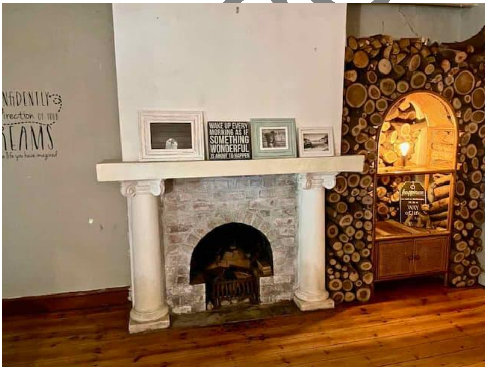
FIGURE 07: c1930's era hearth and similar period mantel supported on precast columns with Ionic capitals matching those on the veranda.
