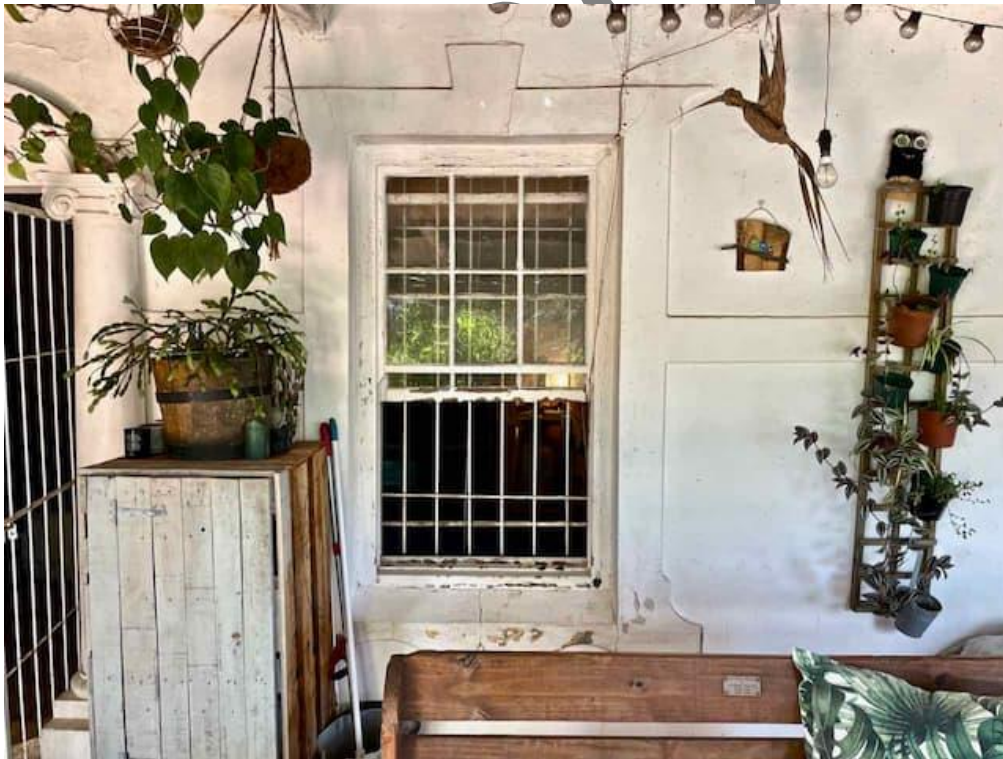
FIGURE 03: Latter 19th/early 20th C small pane sash windows with plaster surrounds.
