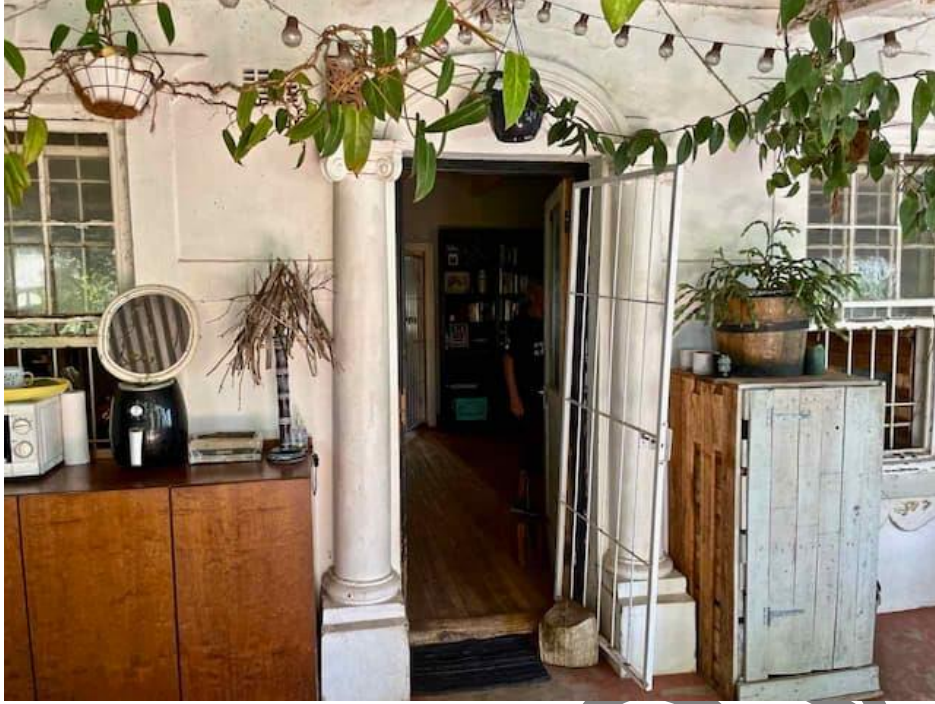
FIGURE 02: Front doorway with flanking c1930's era precast ionic columns and plaster mouldings.
