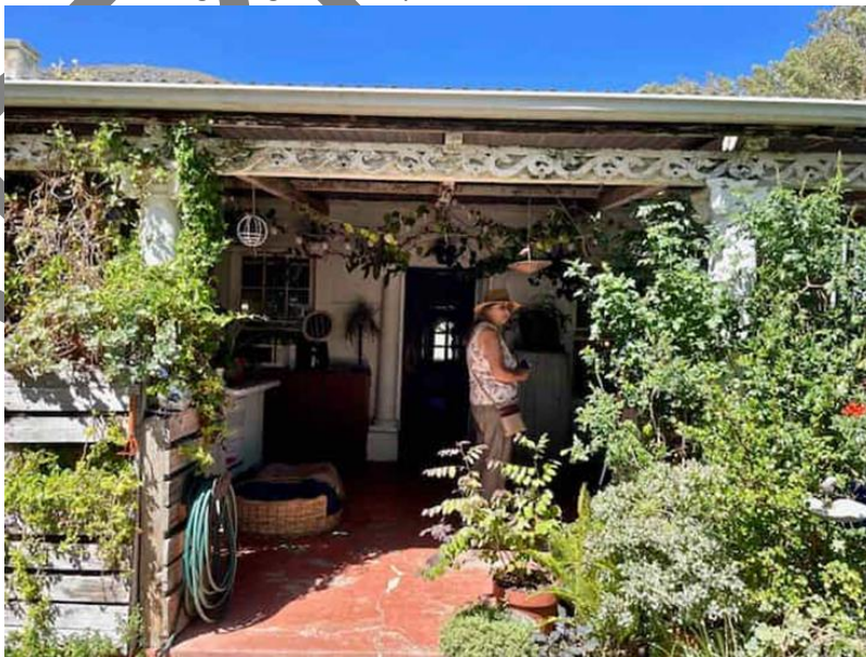
FIGURE 01: Front veranda with recycled timber fretwork applied to the eaves beam.
