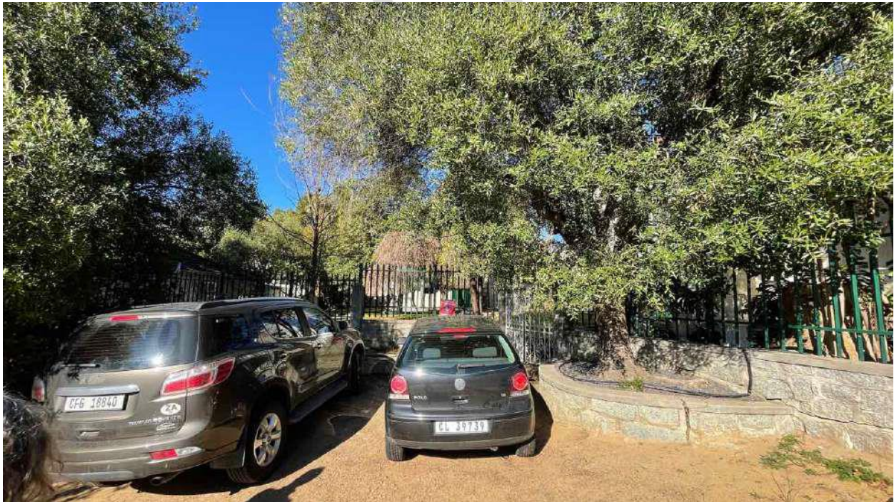
FIGURE 03: Granite pillars and retaining walls that would be displaced by the proposed building. The trees in the foreground would in all likelihood also have to go.
