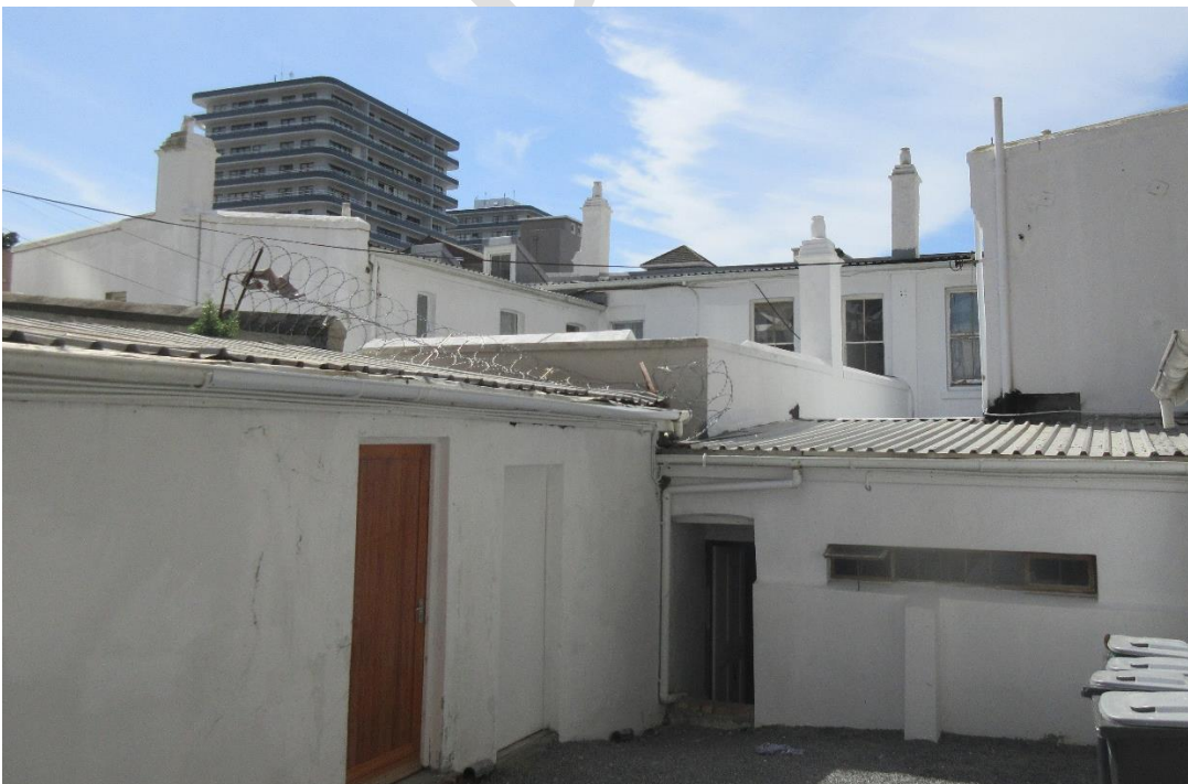
The E-shaped footprint, which allowed lighting and ventilation to all rooms; the roofscape of chimneys, with cast iron mantelpieces internally, and unusually, light scoops over staircases.
