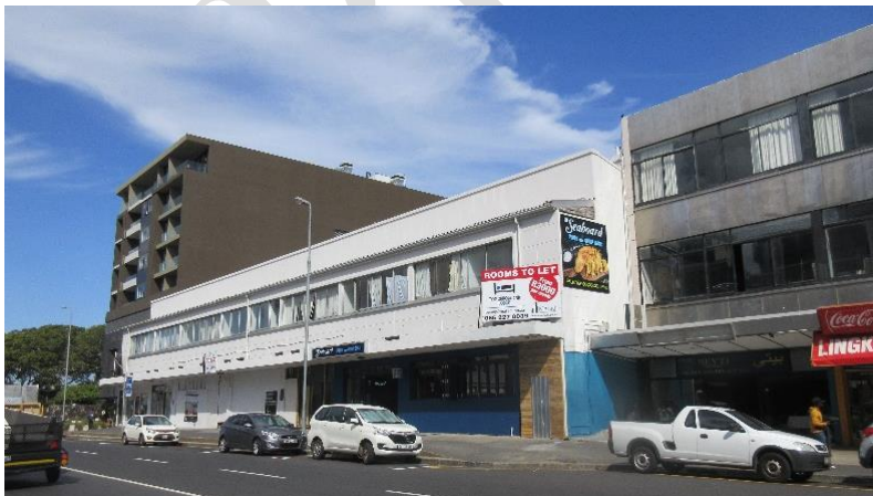
Subject building within its context on south-east side of Main Rd.
