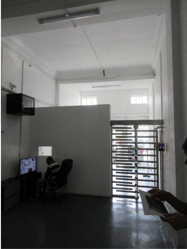
The unusually high floor to ceiling height of the ground floor, with clerestory windows located above the external canopy providing natural light.
