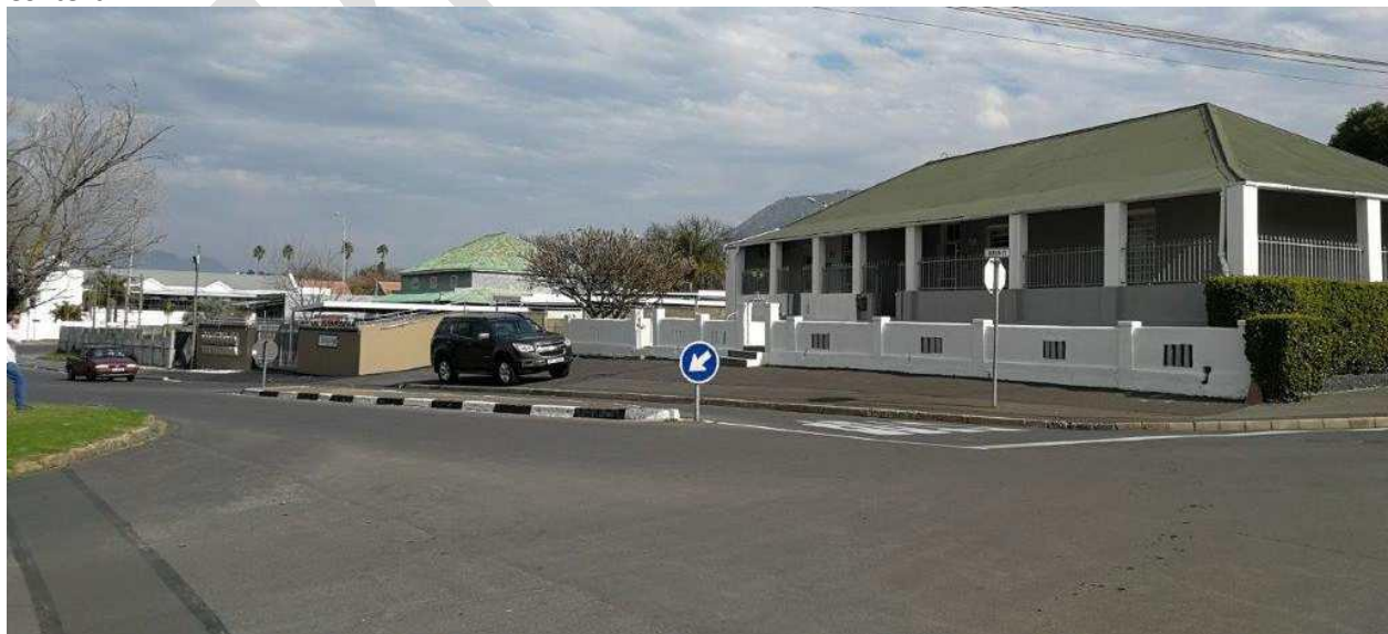
View from corner Berlyn & Bosch Str, showing nearest intact period building, & No 70 behind
