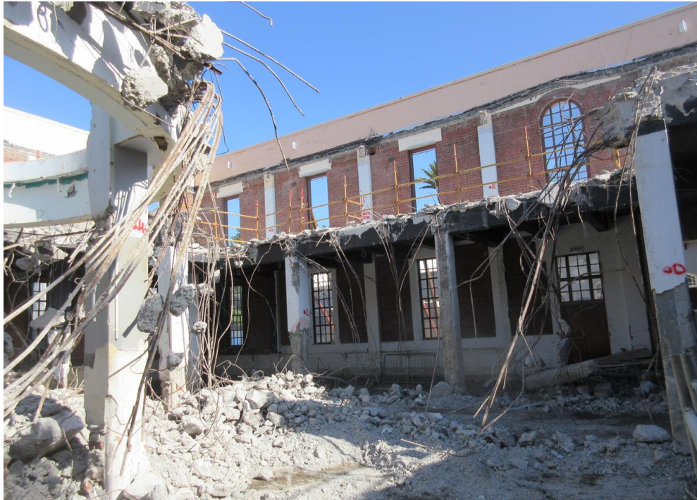
Fig.3 View towards the west wall
