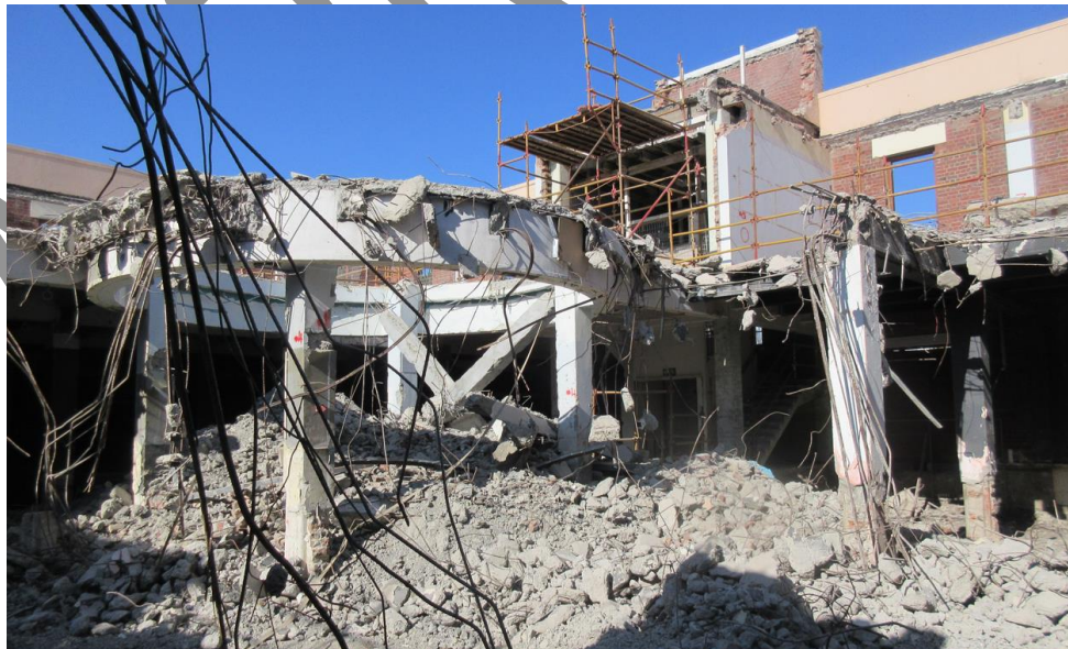
Fig.4 View towards the south wall
